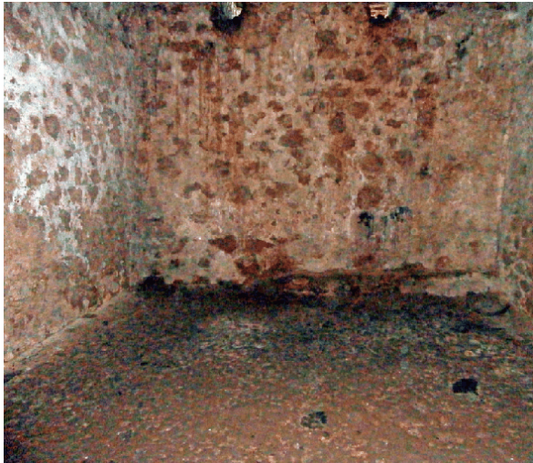
Figure 27: Part of the men cellar Source: Apoh, 2019
